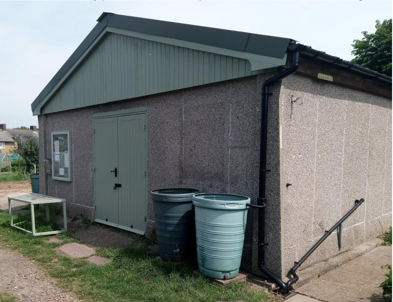
The site 2 newly painted store with repositioned water butts and drainage
