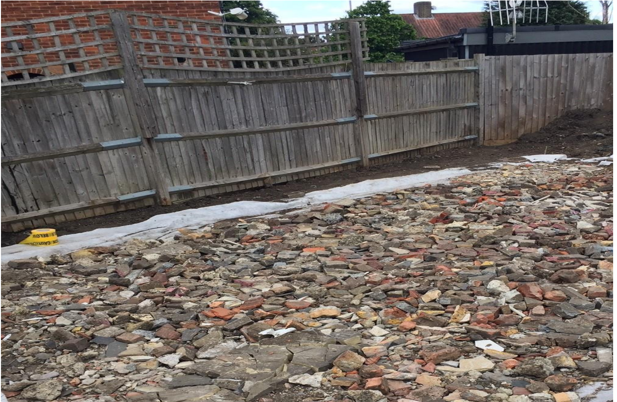
Getting ready for a tea hut on Site 3 – nearly there!
