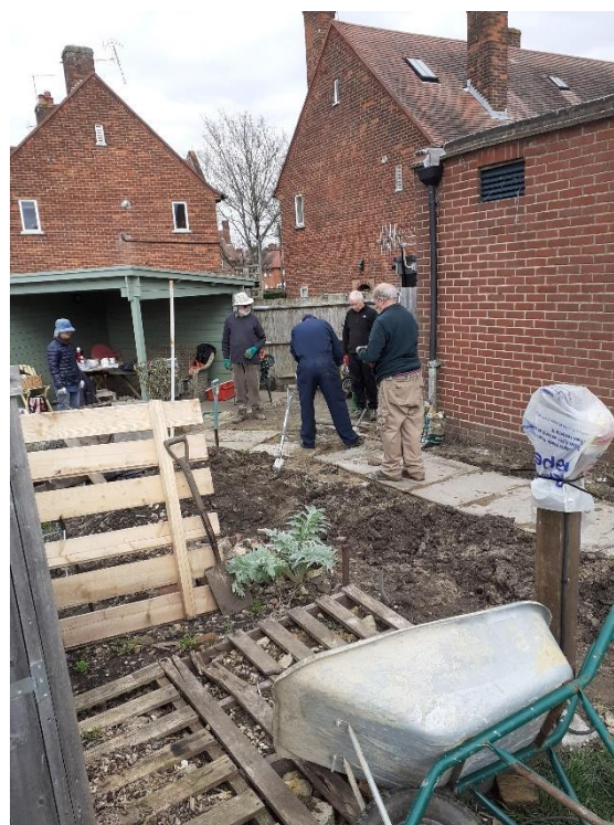
Volunteers laying the path on Site 3
